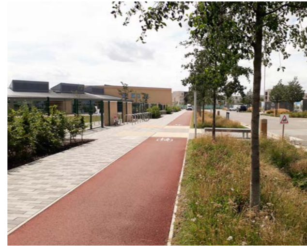
Example of dedicated space provided to cyclists and pedestrians separated from the carriageway with tree planting and sustainable urban drainage.
