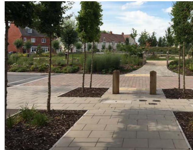
Example of a junction between a street and a footpath where a raised table and textured paving gives priority to pedestrians
