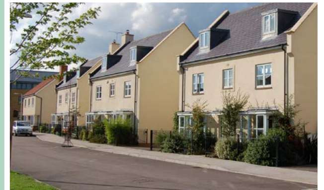
On plot parking to the side.
