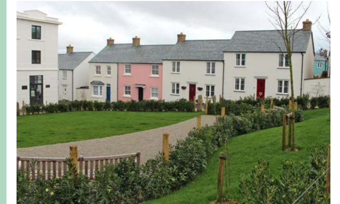
Consistent approach to character through materials, building form and building set back. Planted boundary to public space. Coloured render is used to add interest.
